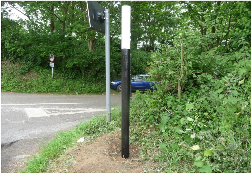
Figure 4 Cleaned and Painted Post
