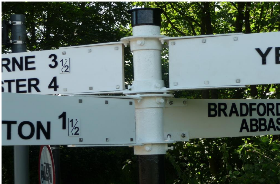
Figure 9 Reassembled Components on Pole
