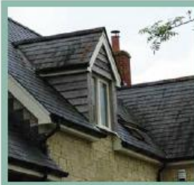
Gable wall dormer with side hung casement window
