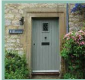
Plank door set within a stone dressing
