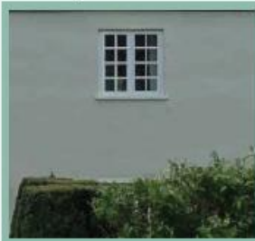
Light coloured render over rubble-stone walls
