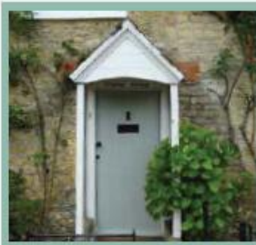
Timber gable porch canopy with two wooden posts
