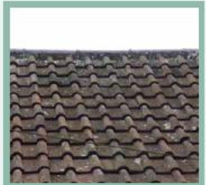
Double Roman interlocking roof tiles
