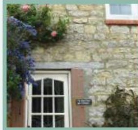
Leadlight glazing set in door, timber lintel and brick cills
