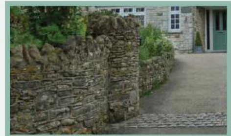
Stone wall with lime mortar topped with larger 'cock and hen' cap stones.
