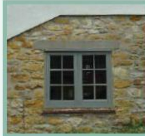
Painted timber casement window with stone lintel
