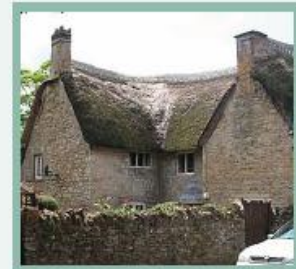
U-plan thatched roof with gable ends
