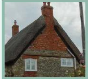
Gable end thatched roof with red brick chimney stack
