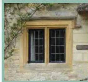
Iron casement window with chamfered stone mullions
