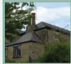
Slate hipped roof with integrated side range
