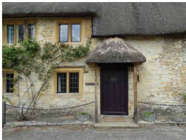
Figure 22: Chantry Cottage: Grade II listed detached cottage featuring a rubble-stone wall, thatched gable roof, thatch porch canopy with wooden posts and windows with hollow-chamfered stone mullions and iron casements.
