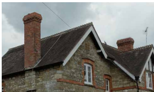
Figure 54: Example of a overhanging verge, exposing the purlins and the outer rafter.
