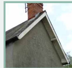
Overhang verge with a soffit of diagonal timber boarding
