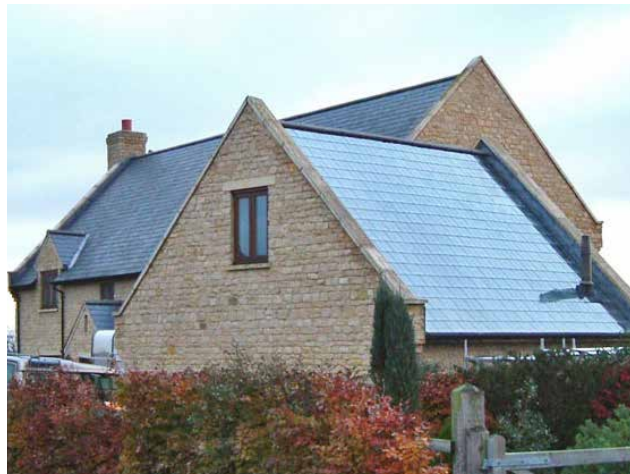
Figure 57: Solar panels should be integrated into the design of buildings from the outset. This example of a new home in a Conservation Area shows how the panels can mimic the appearance of traditional slate roofs.
