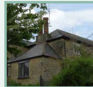
Slate hipped roof with integrated side range
