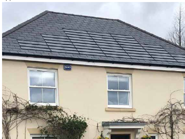
Figure 58: Use of shingle-like solar panels on a slate roof, with the design and colour of the solar panels matching those of the adjacent slate tiles in Lingfield, Surrey.
