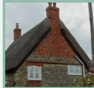
Gable end thatched roof with red brick chimney stack
